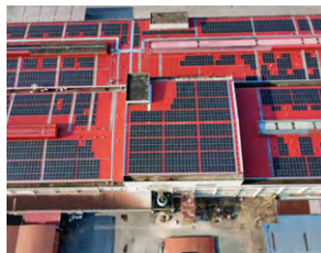
Li Quan Plant
